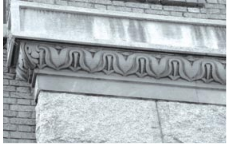
A feature of the Grinnel building.
